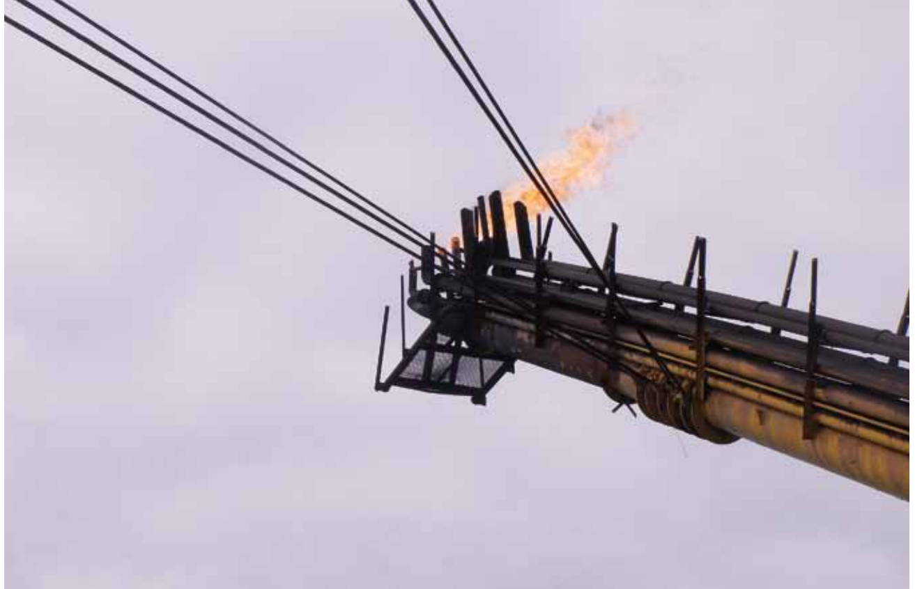
Gas flare on an oil and gas platform, Cook Inlet, Alaska.
